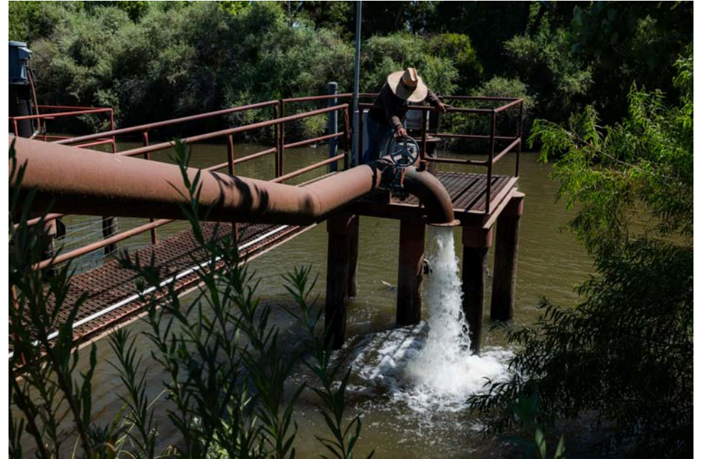
A “ditch rider,” a person who inspects irrigation systems and distributes water to farmers, adjusts the return flow to a Delta waterway.
