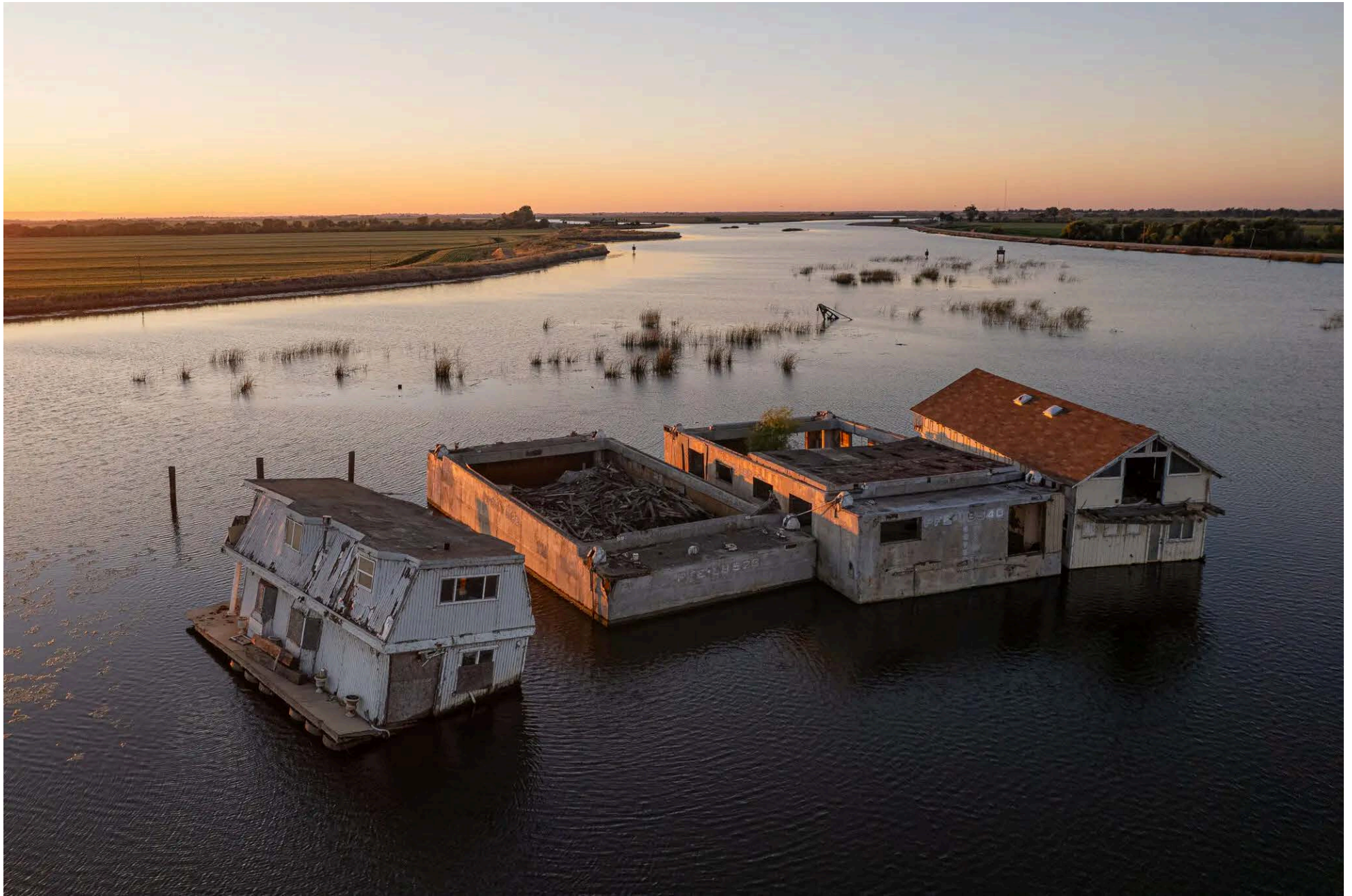
Remnants of the abandoned Herman and Helen's Marina on 8 Mile Road outside of Stockton.
