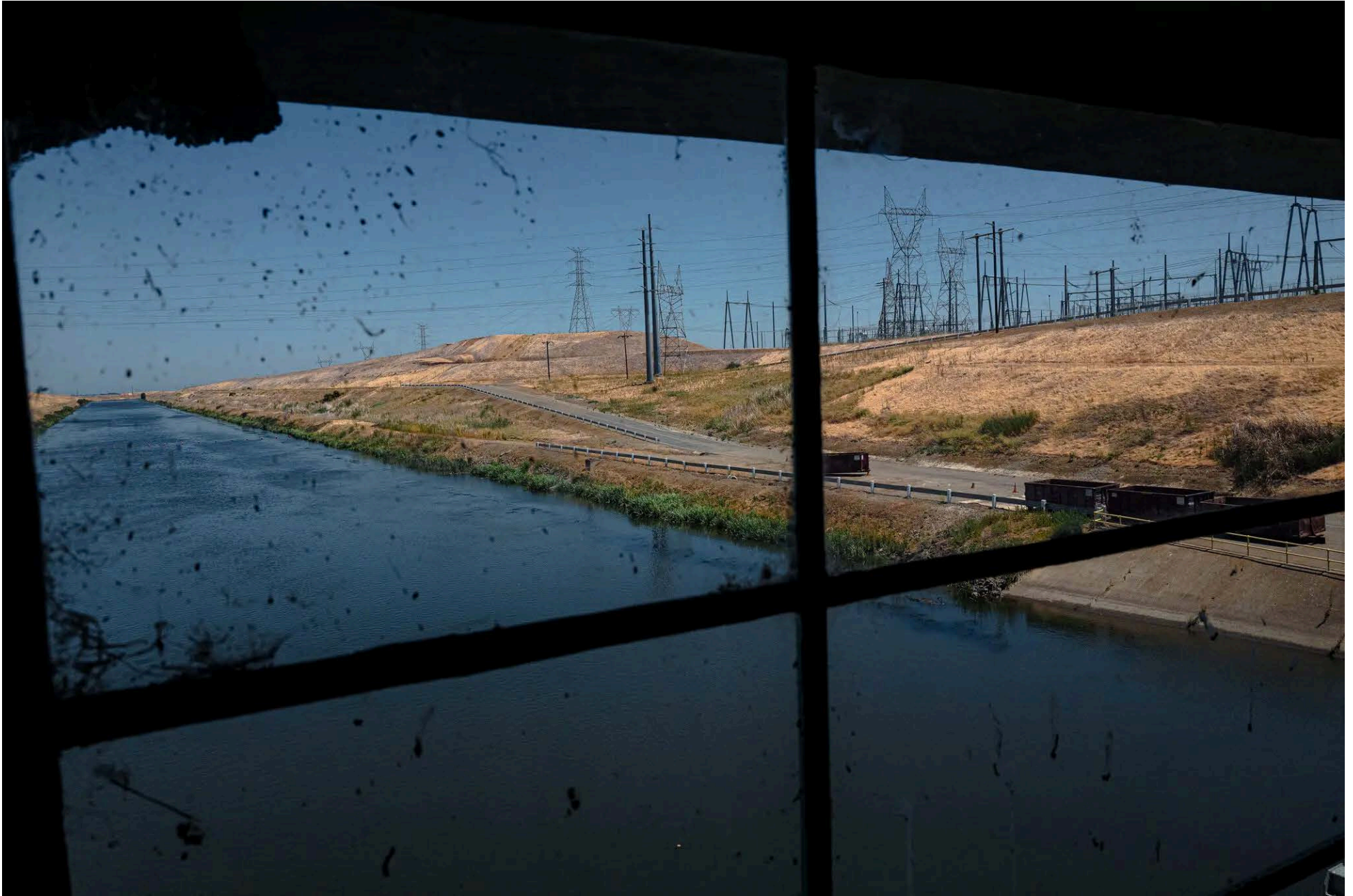
A view of water entering the Jones Pumping Plant in Byron. The plant takes water from the Delta and sends it into the Delta-Mendota Canal.
